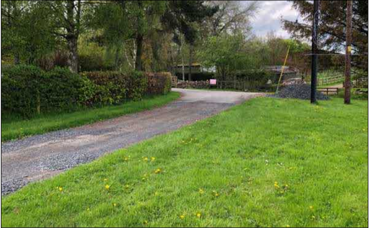
Figure 13. Standard of access track formation as it passes 'The Roost'. Source: Ferguson Planning Site Visit.
