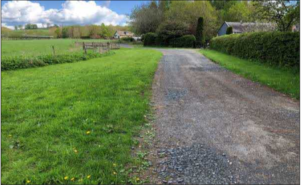
Figure 12. Standard of access track formation to the east of 'The Roost'. Source: Ferguson Planning Site Visit.
